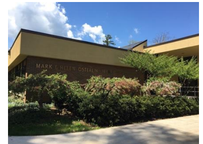
Osterlin Building – SE Exterior
