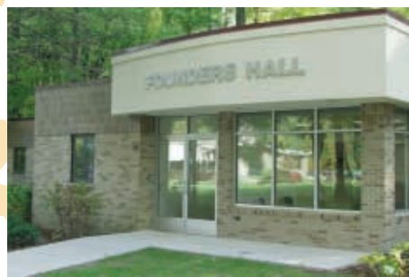
College Relations is back on main campus in the renovated Founders Hall.
