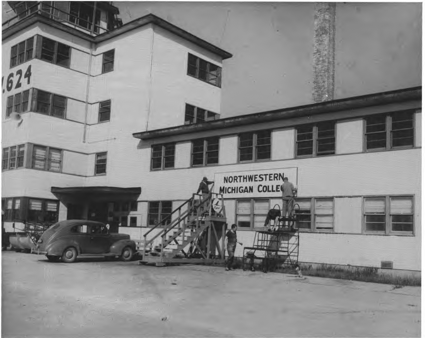
Volunteers erecting a sign on the first home of the College
