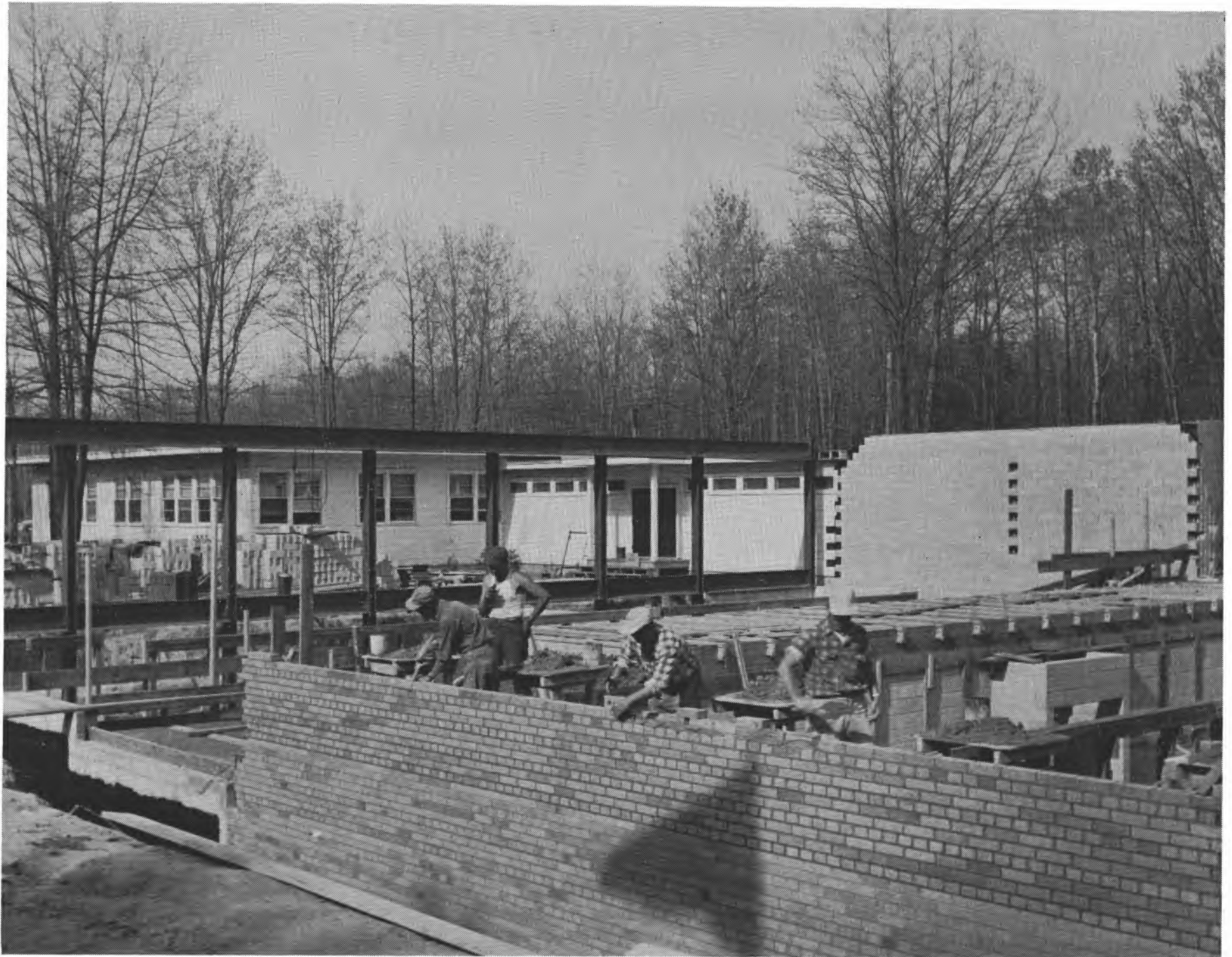
Construction of the Administration Building
