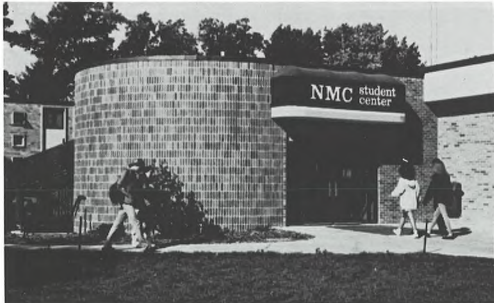
Student Center renovation
